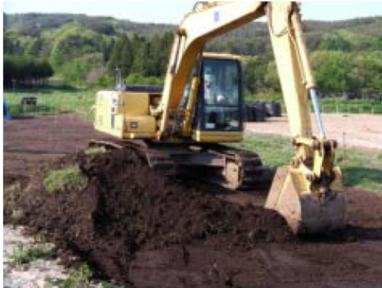
Stripping topsoil method
